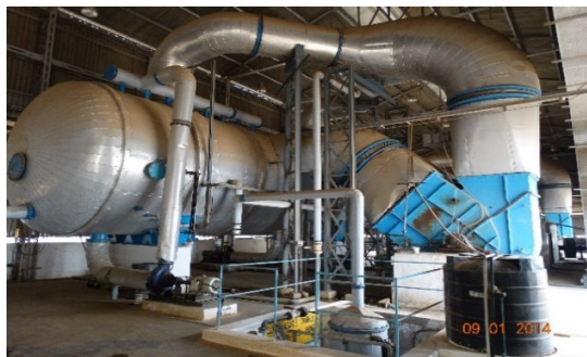
MVR-Evaporator
