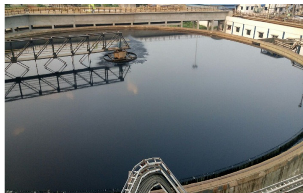
Primary Sedimentation Tank
